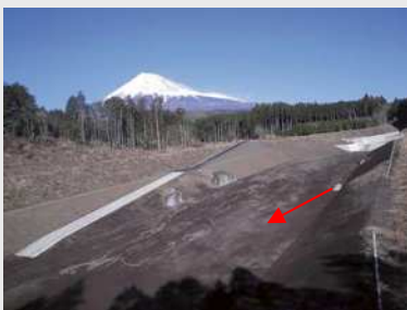
Sand retention works
