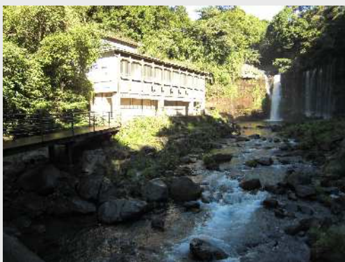
Before Buildings on the waterfall basin
