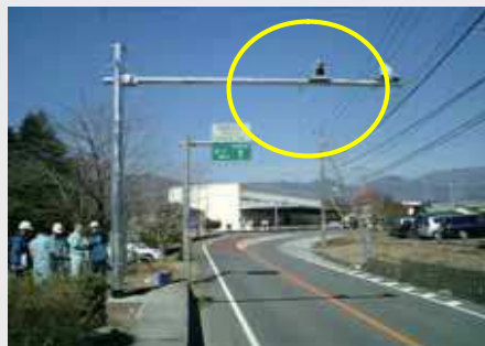
Installation of surveillance cameras as a measure to prevent illegal waste dumping
