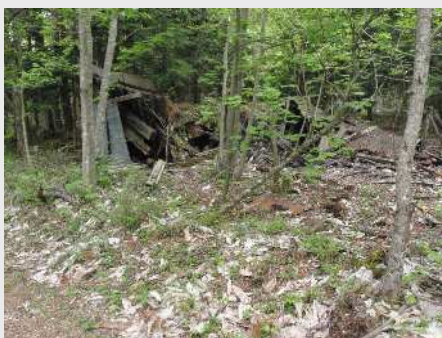
Dilapidated mountain hut
