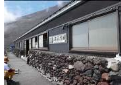
A mountain hut designed on the model of traditional Iwaya (rock-covered house)
