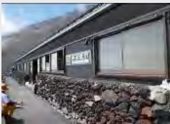
Exterior appearance of a mountain hut that retains the atmosphere of a rock cave
