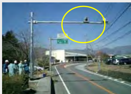
Installation of surveillance cameras as a measure to prevent illegal waste dumping
