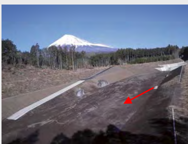
Sand retention works
