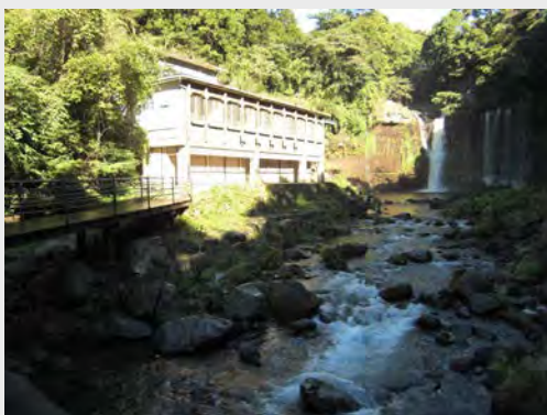
Before Buildings on the waterfall basin
