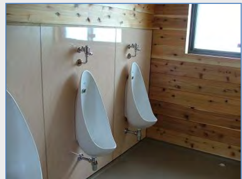
All the toilets have been replaced with environmentally sensitive toilets (human waste issue has been solved.)
