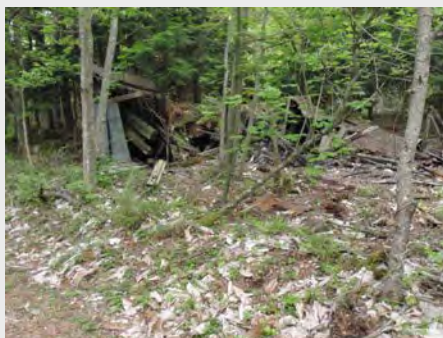
Dilapidated mountain hut
