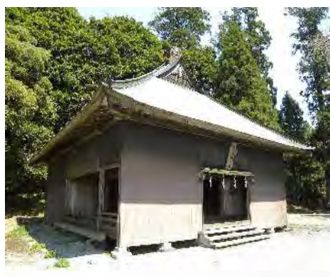
Murayama Sengen-jinja Shrine - Pre-Dainichido Repairs
