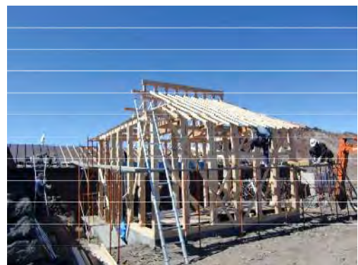
Rear Shrine Main Hall Under Renovation
