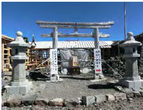
Rear Shrine Under Repair
