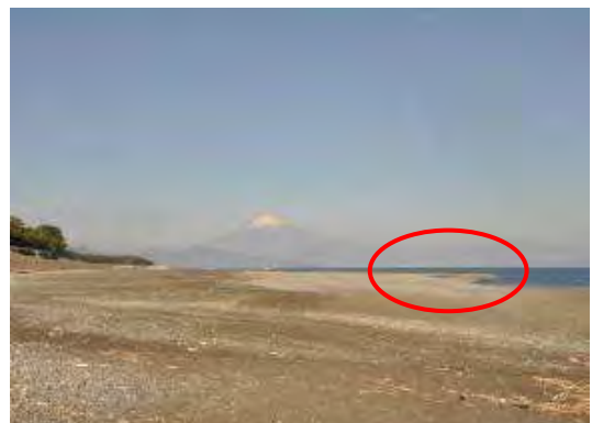
< L-shaped Protruding Dams 20 Years Later >
