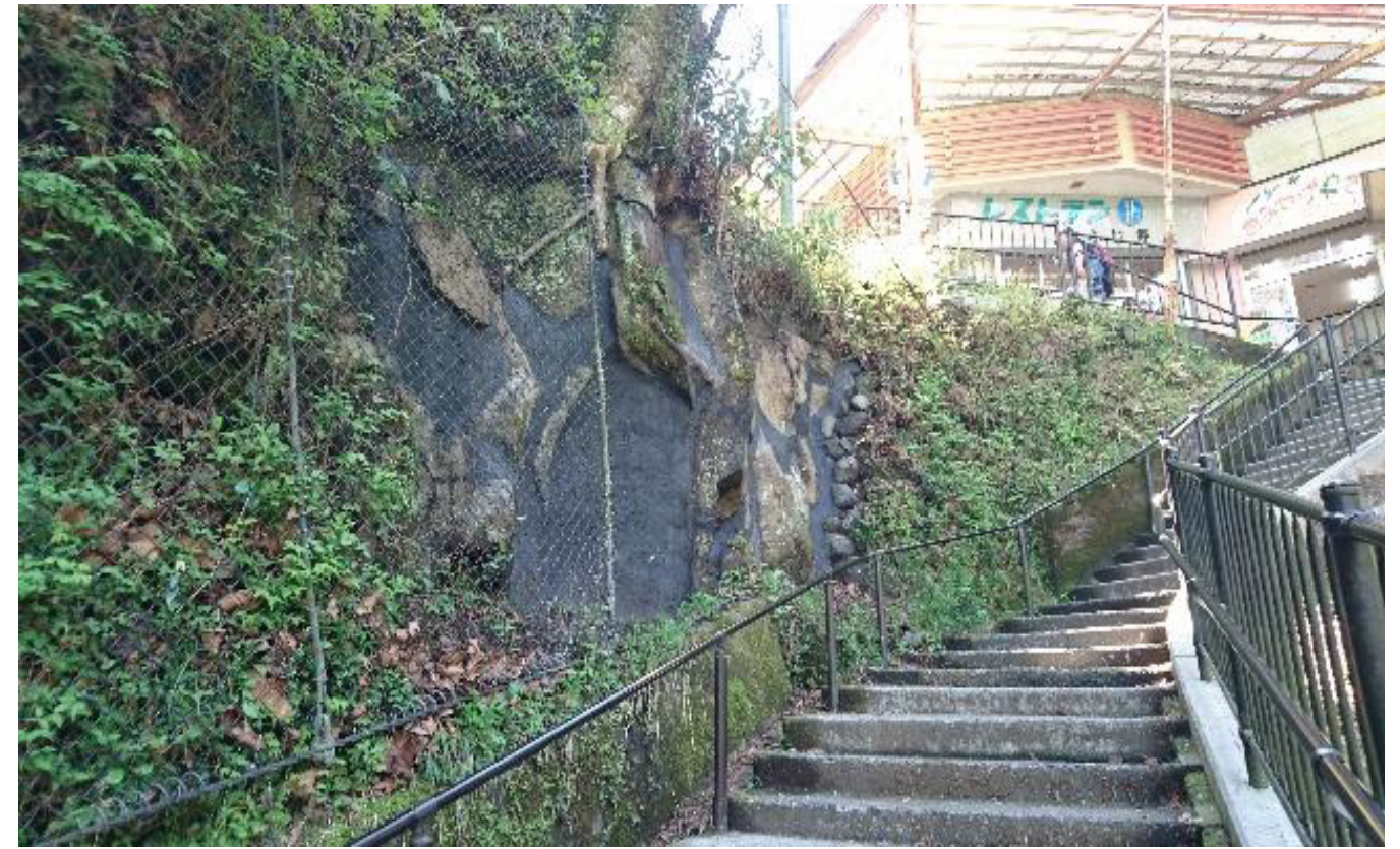
Reinforcement of the bedrock along the steps
